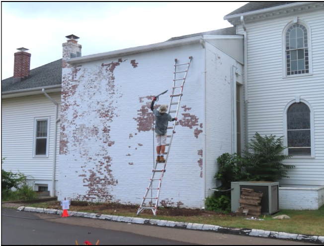
LEFT: July 14, 2025. Chris Gann power washing the mural wall after scraping off all the peeling paint. The hedge at the base of the wall has been removed.
